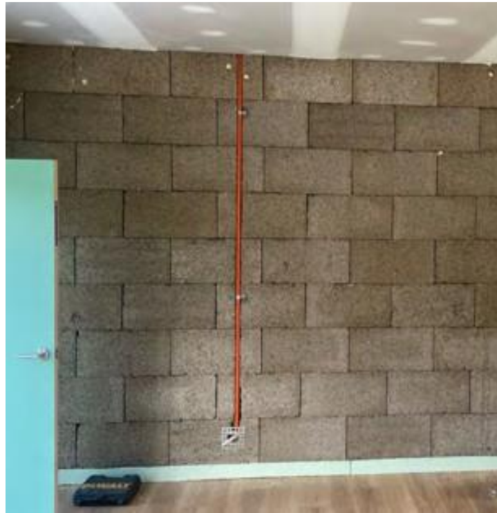
Figure 104 - Embedding service ----- and -----Figure 105 - Embedding ducted services
