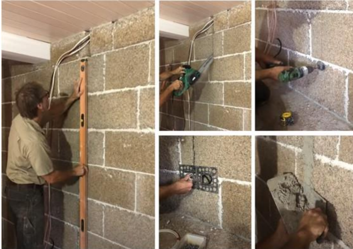
Figure 106 - Embedding services into a HempBLOCK wall
