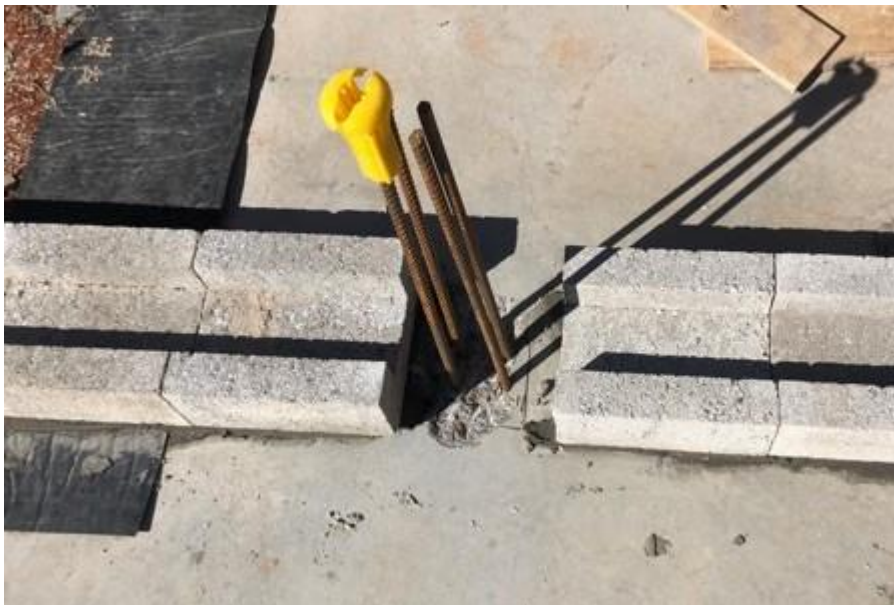
Figure 30 - Concrete starter blocks
