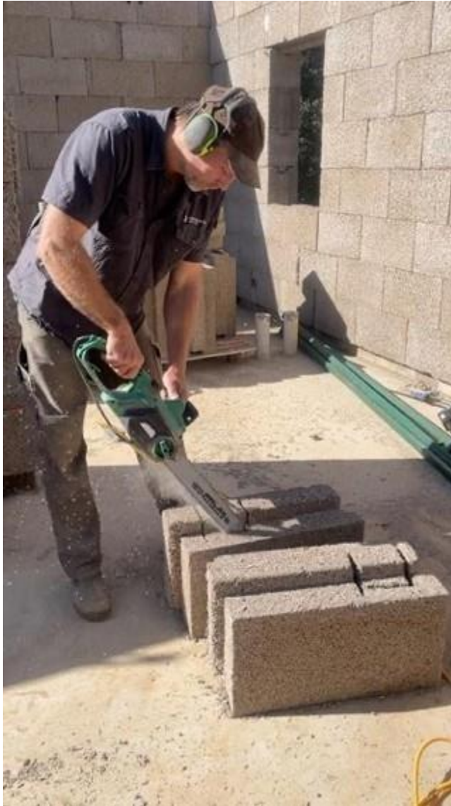
Figure 33 - Cutting a column hole
