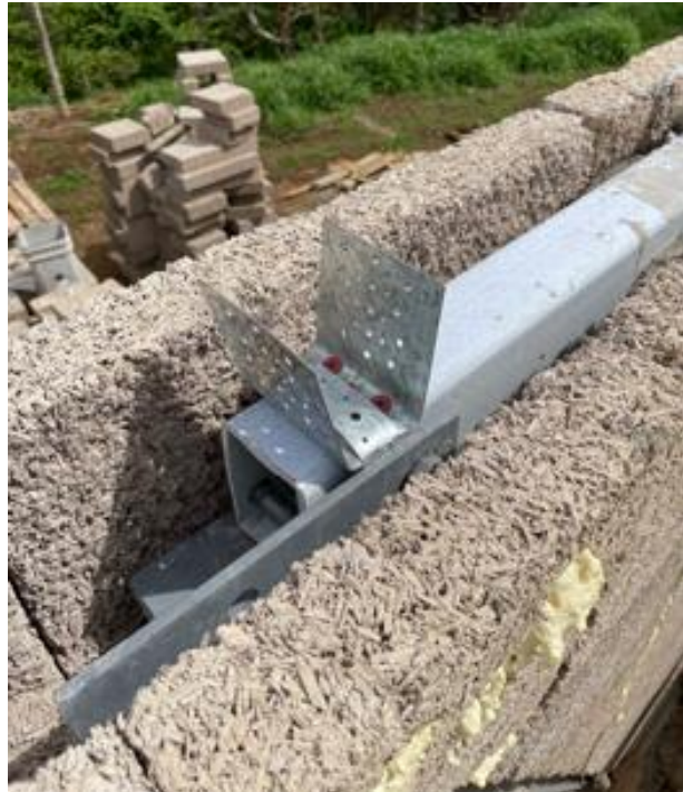
Figure 75 - Burman roof anchor brackets
