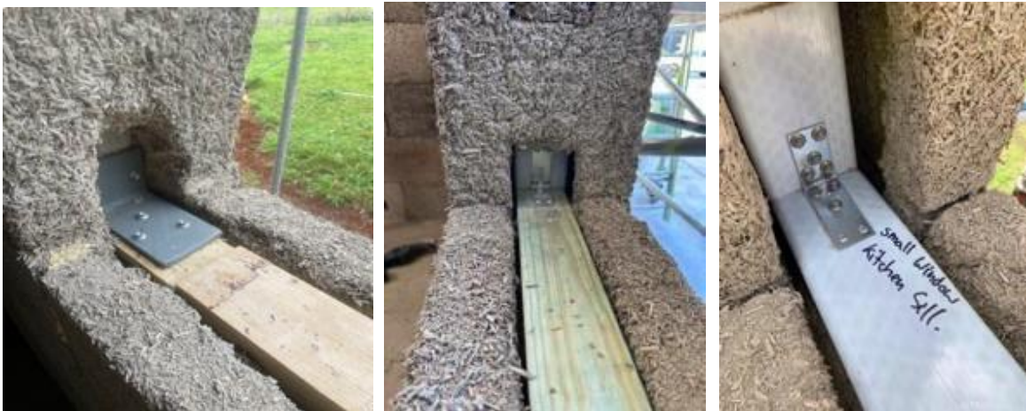
Figure 60 - Installing windowsills
