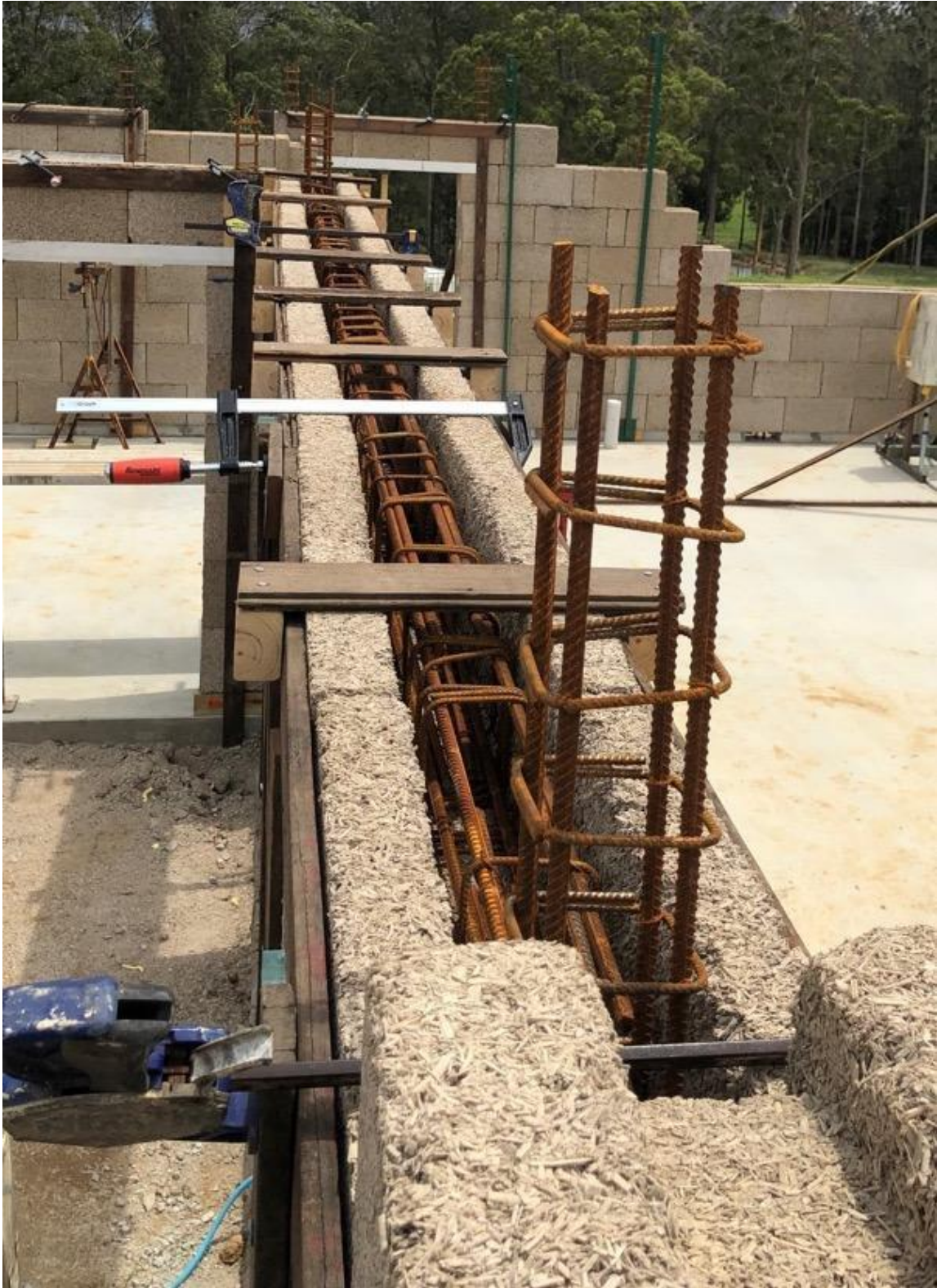
Figure 85 - Bracing a steel reinforced concrete system before casting
