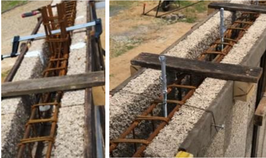
Figure 98 - Ring beam cages
