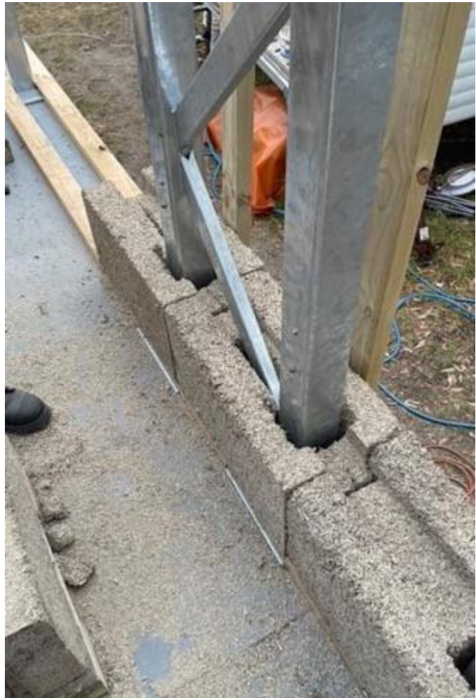
Figure 28 - K-brace installation
