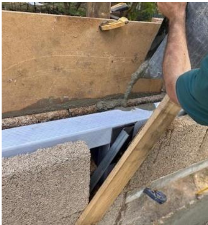
Figure 76 - Mixing and placing a perlite-cement mix
