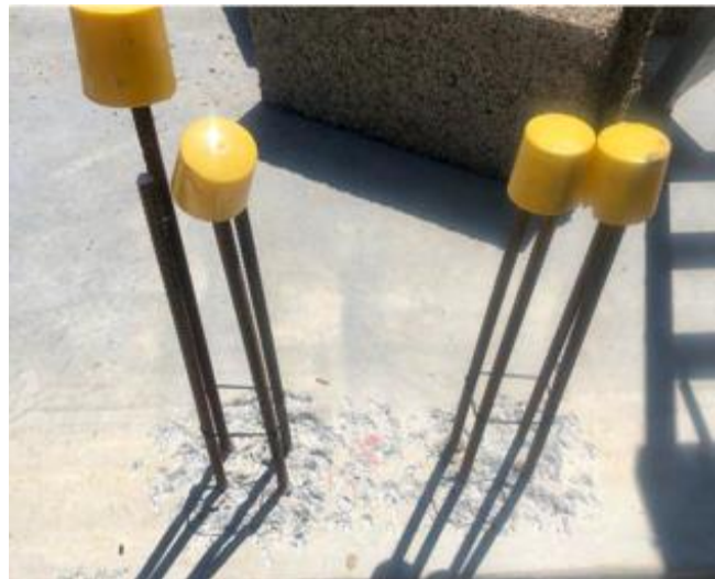
Figure 24 - Starter bars
