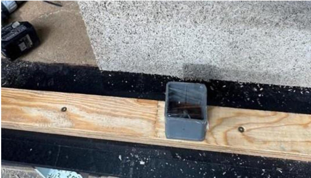
Figure 20 - Tongue, stanchion on timber floor
