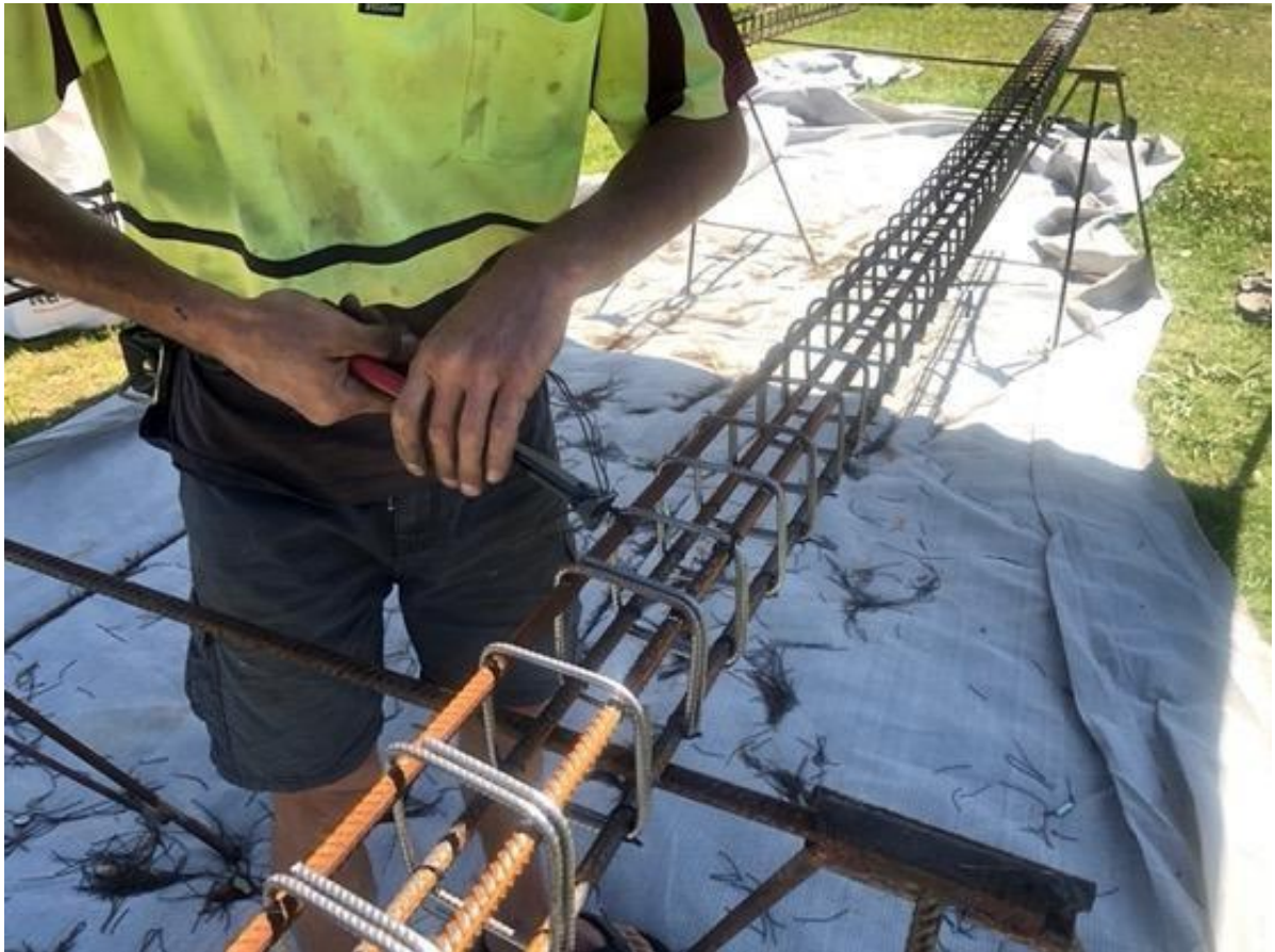
Figure 77 - Making steel cages
