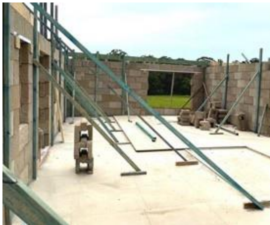
Figure 72 - Safety struts on incomplete walls
