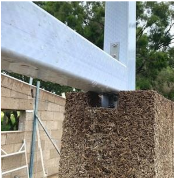
Figure 64 - FRP window lintel supporting blocks
