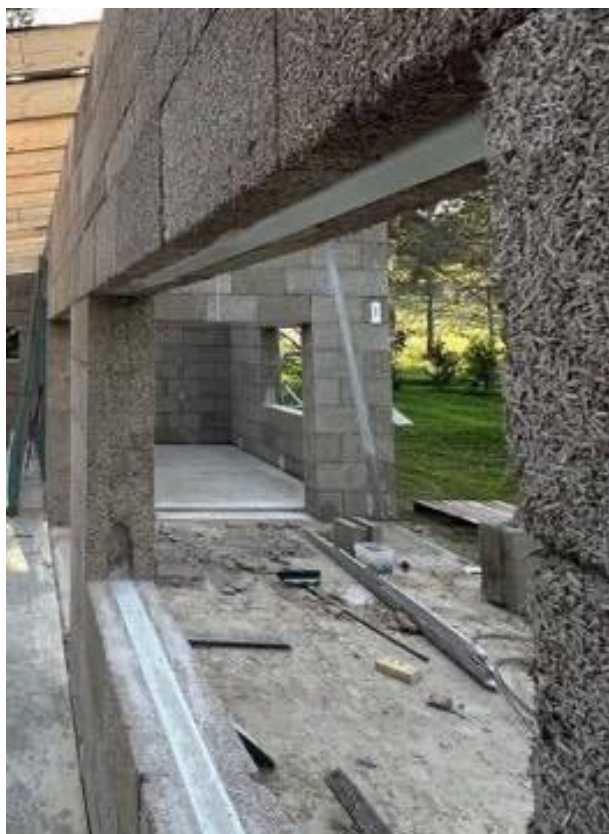
Figure 65 - Lintel (header) supporting blocks
