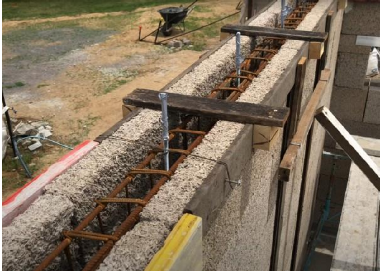
Figure 86 - Bracing a steel reinforced concrete system before casting
