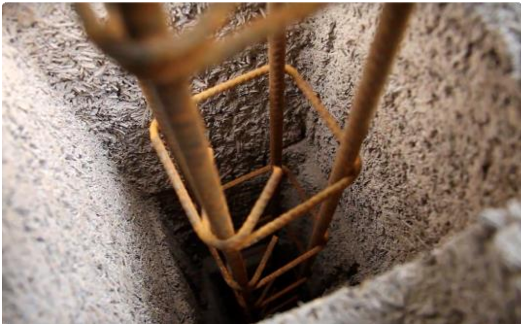
Figure 80 - Steel cage (10mm rebar only)
