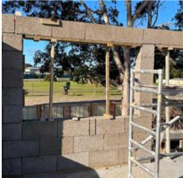
Figure 71 - Placing U-blocks
