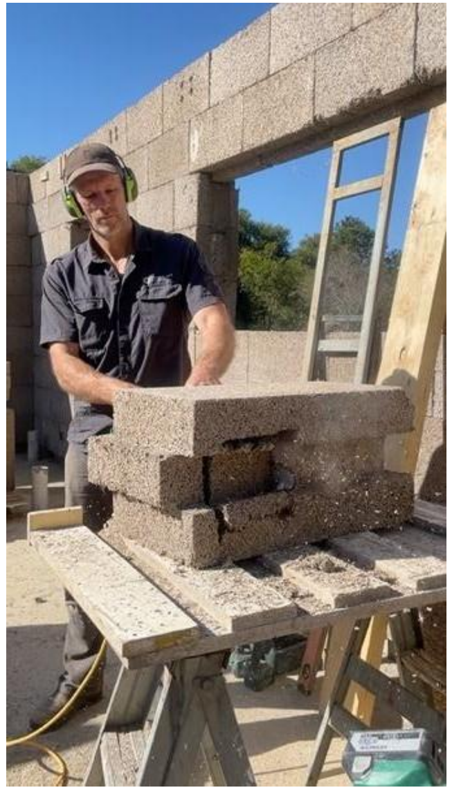
Figure 33 - Cutting a column hole
