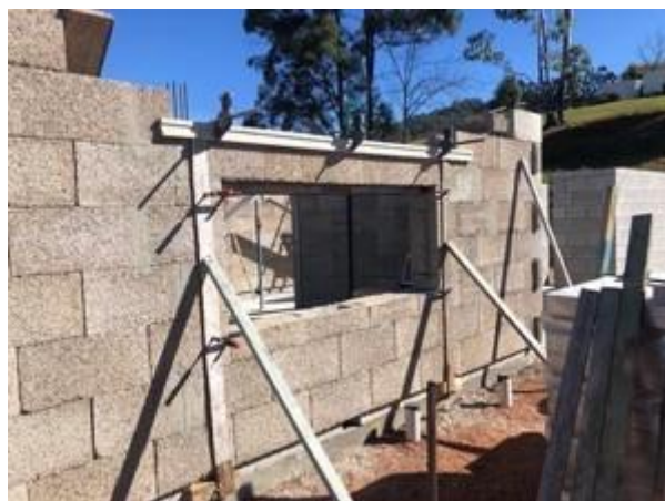
Figure 72 - Safety struts on incomplete walls
