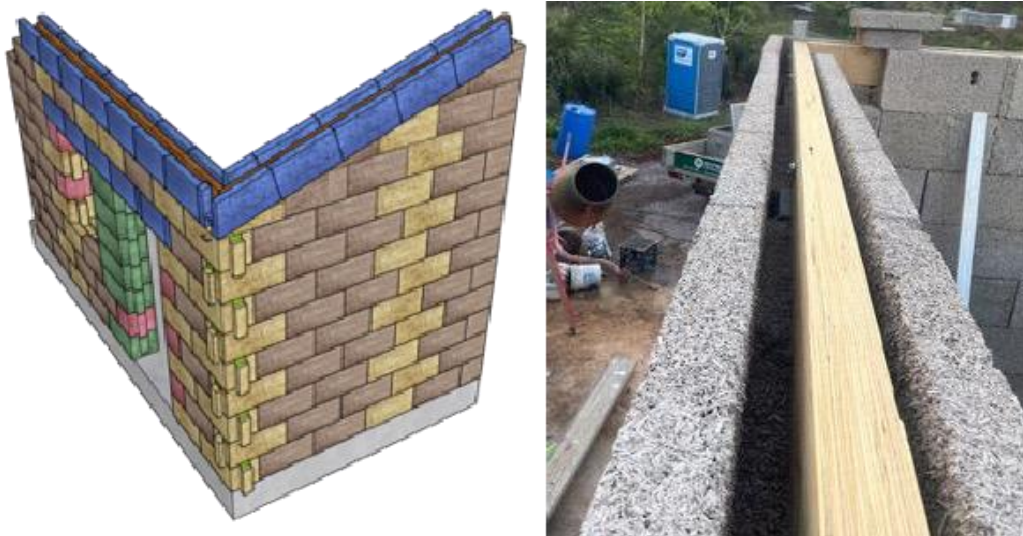
Figure 15 - Bond beams before perlite infill
