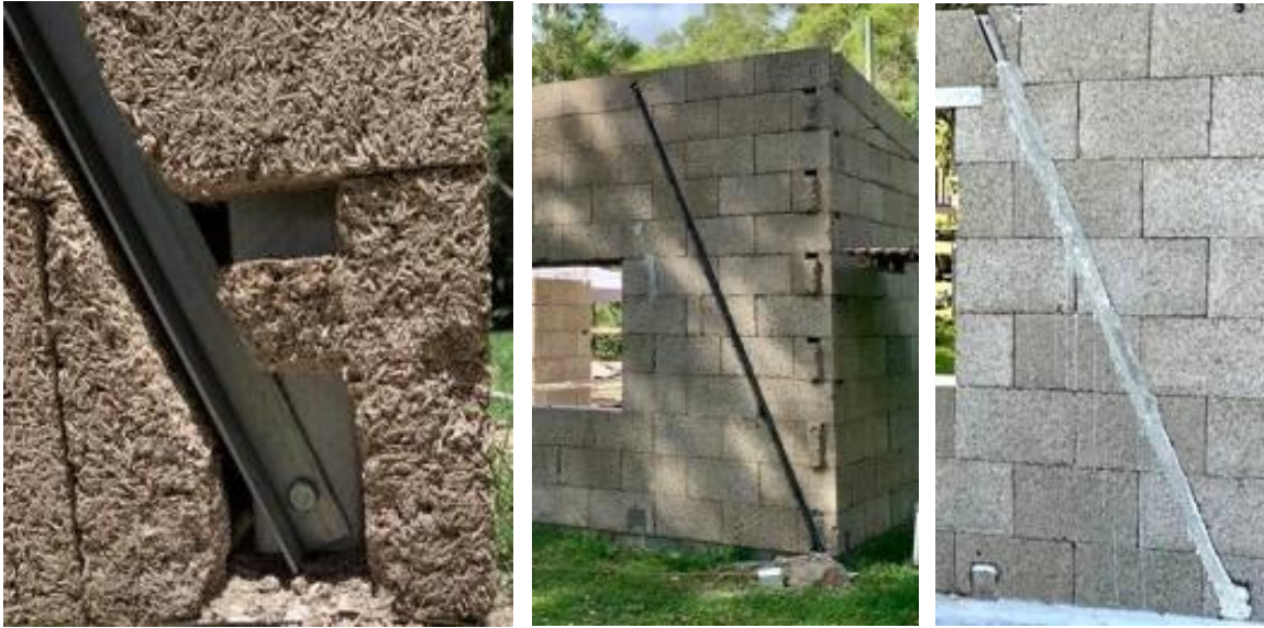
Figure 59 - A diagonal braces
