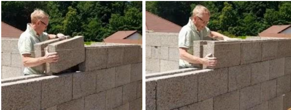
Figure 48 - Stacking blocks
