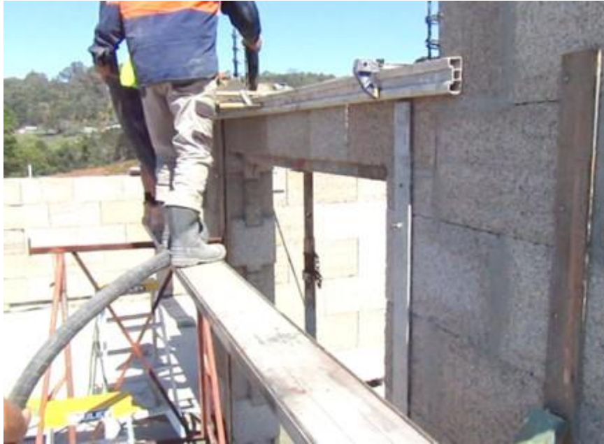
Figure 89 - Casting the lintel
