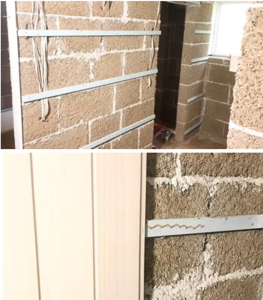
Figure 112 - Battening out and cladding
