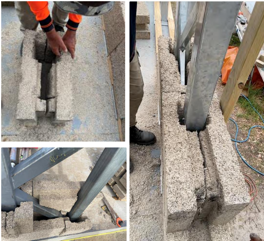
Figure 51 - Encasing a K-brace
