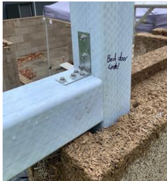
Figure 64 - FRP window lintel supporting blocks
