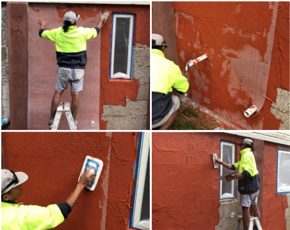
Figure 111 - Rendering the first layer with mesh reinforcement
