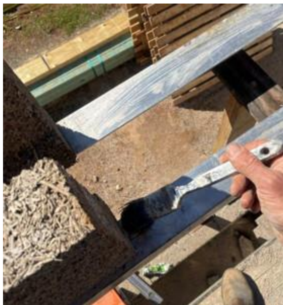
Figure 69 - Applying releasing agent
