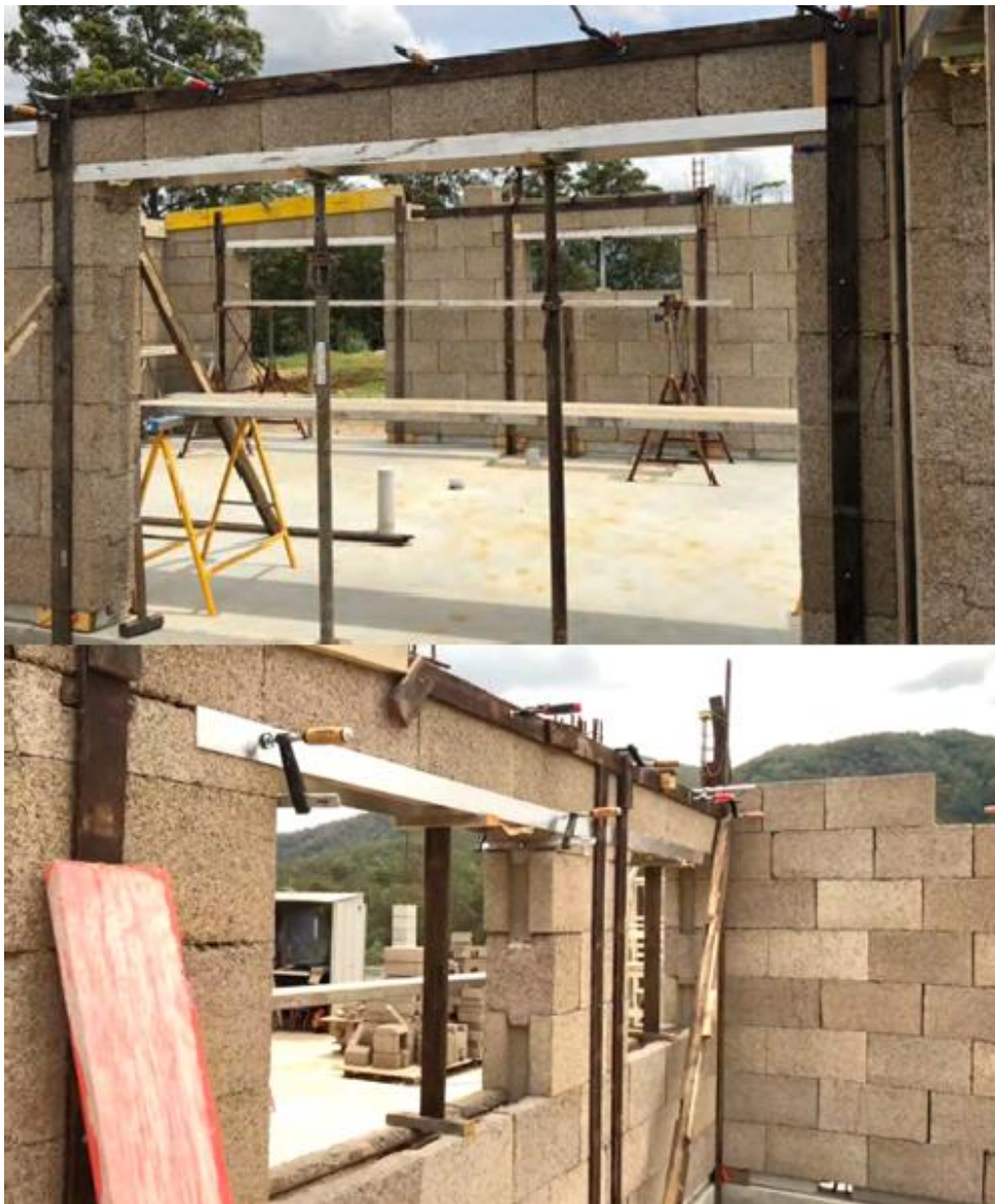
Figure 84 - Bracing a steel reinforced concrete system before casting
