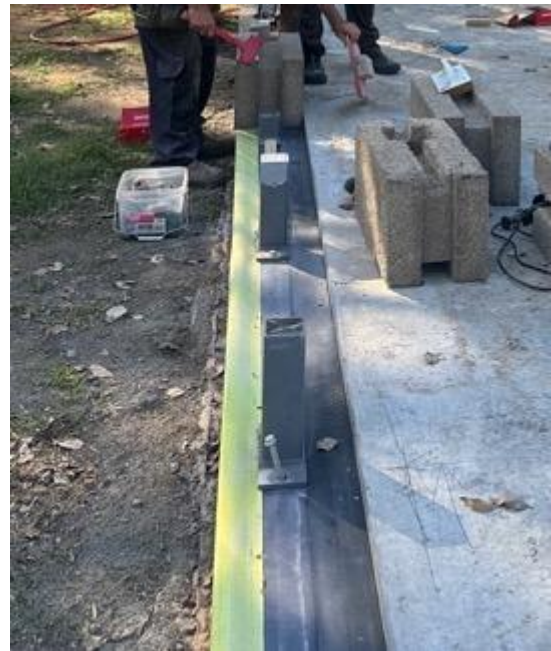
Figure 26 - Steel foot (stanchion) installation
