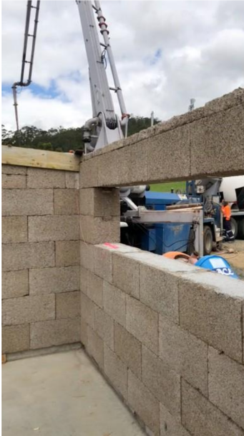
Figure 98 - Casting concrete with a concrete boom pump
