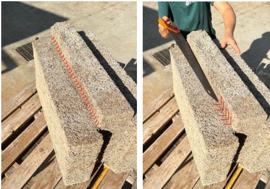
Figure 6 - Shaving the edge of the tongue
