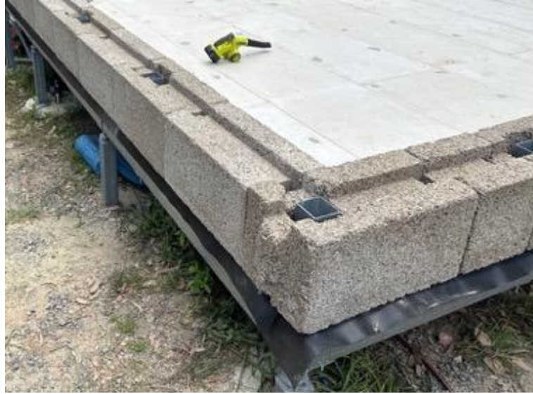
Figure 19 - Fire resistant magnesium board floor
