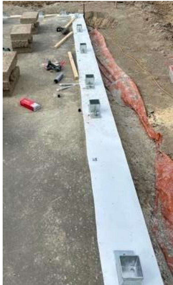
Figure 25 - Waterproofing and termite proofing in one
